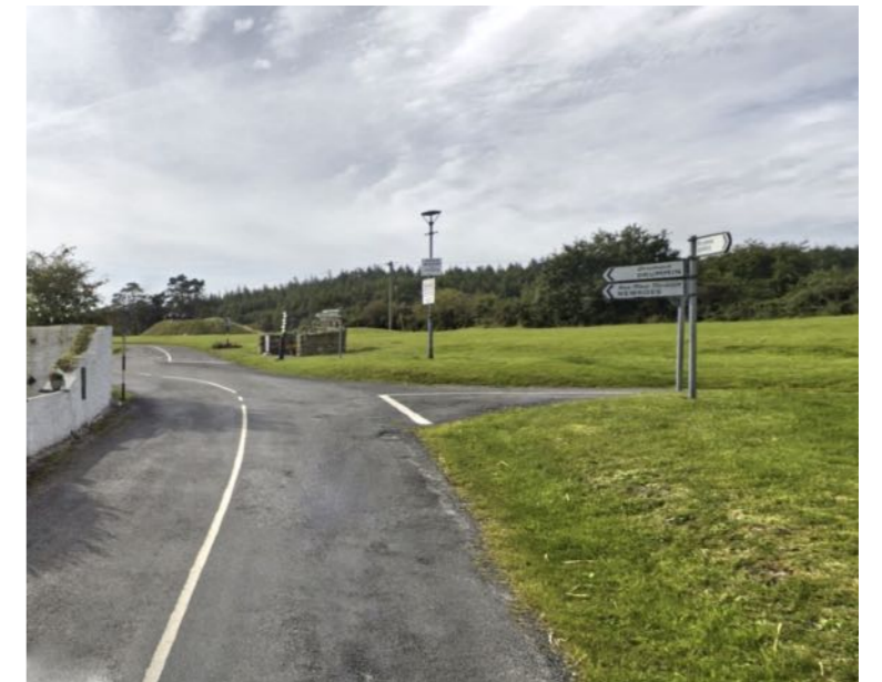
Figure 25 - L3008 Village Green Signposting
