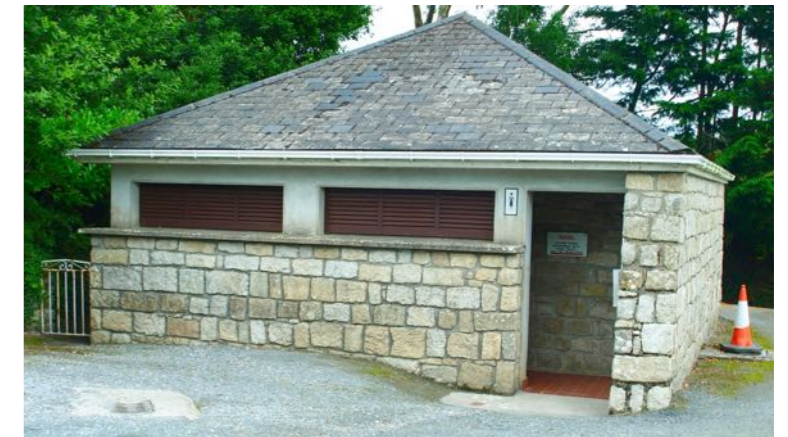
Figure 11 - St. Mullins Public Toilets
