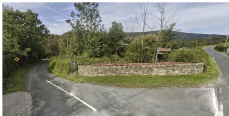
Southern Entry L3008 (Junction with L30083)
